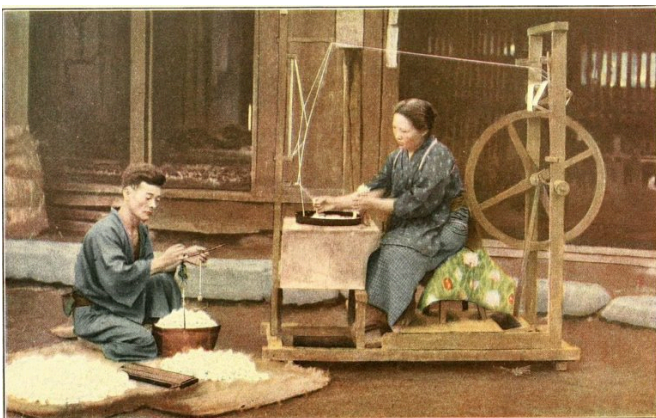
Reeling silk by hand in Japan, from Silk: its origin, culture, and manufacture (1911). Internet Archive Book Images, Flickr, no known copyright restrictions.
